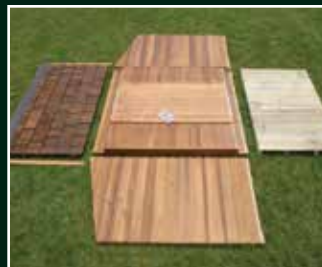
LAY OUT PRE-MADE PANELS
