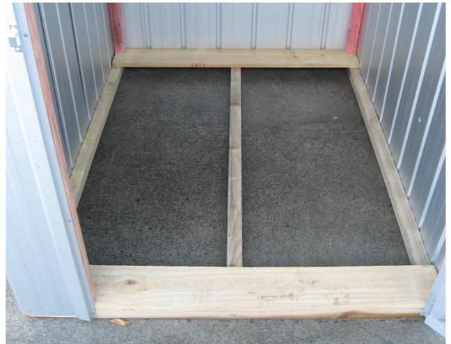
**Step 3:** Lay out remaining Floor Boards. You may need to cut the last Board to correct width using Skill saw. Nail in each Floor Board, two 50mm nails each end and two into Floor Joist.
