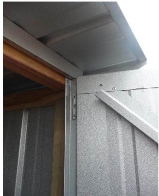
**Step 3:** Close door and check it fits correctly. If not, drill out rivets and make necessary adjustments. Fit remaining rivets to all three hinges.
