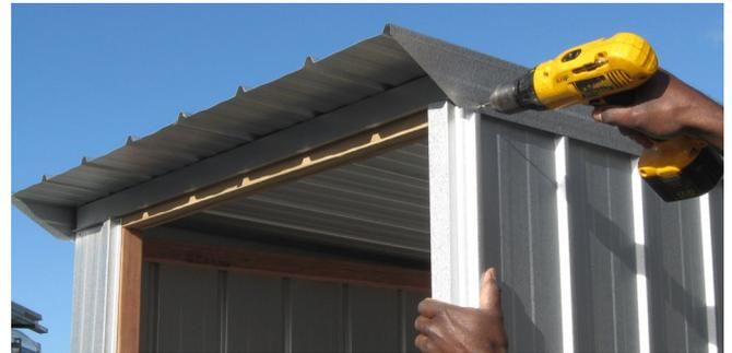
**Step 3:** Line up ribs on the roof with ribs on the walls. While someone holds the Front Plate straight, predrill using a 3.5mm drill bit and screw the roof to Top Plate using one 55mm Roofing Screw on each rib. (Outside ribs do not need to be fastened). Repeat at the back. Note: a string line can be used to make this easier.
