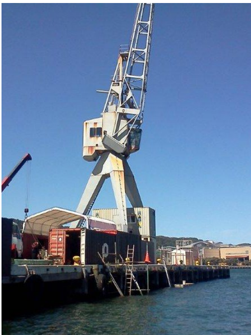
Substantial wharf repairs
